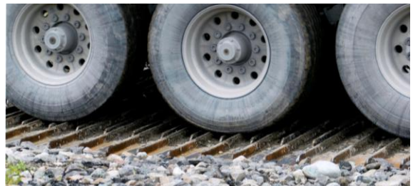
STABILIZED CONSTRUCTION ENTRANCE - RUMBLE STRIP
